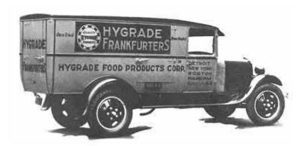
Finally Ford introduced a longer wheelbase Model AA chassis on June 9, 1930. The 157" chassis, which eliminated the need for aftermarket slip-on frames or cut-frame extensions proved very popular with freight haulers and movers.
